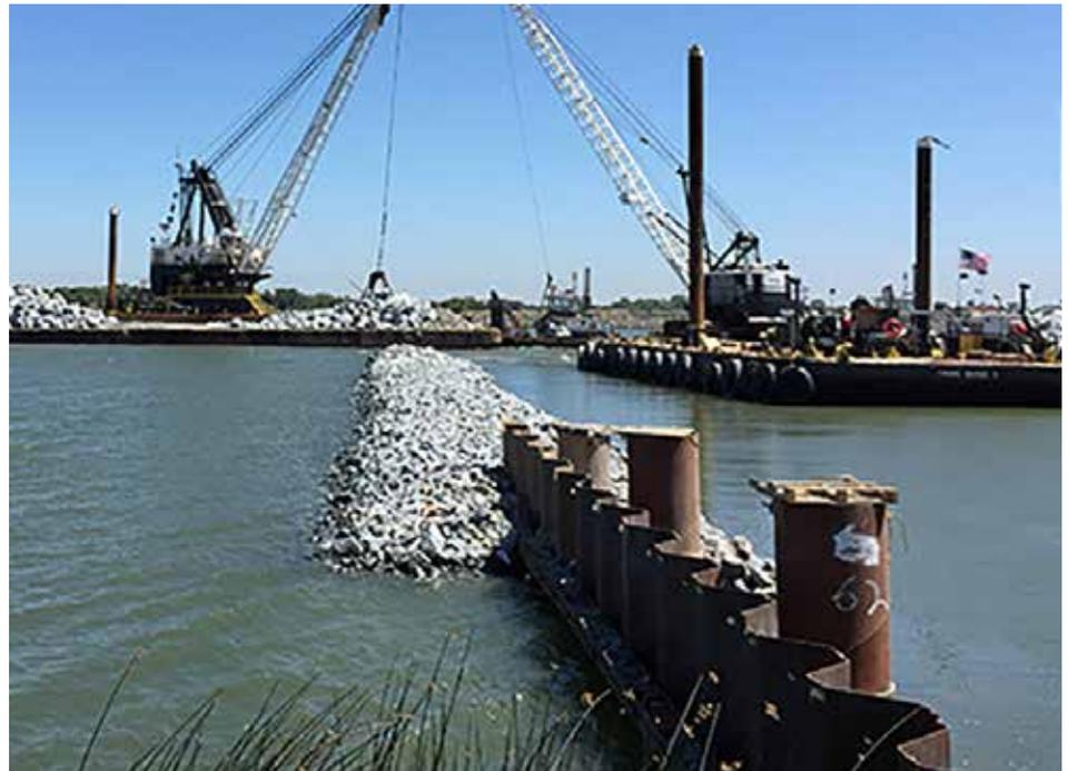
*“The barrier worked by preventing salinity to reach the central Delta... We were able to save about 90,000 acre-feet in upstream reservoirs for the last quarter of 2015 and for fish releases.”*
